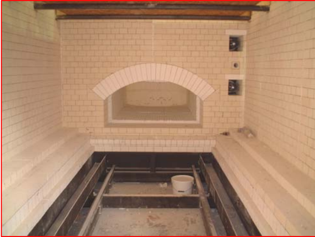
Internal brickwork & inlet into Afterburner
